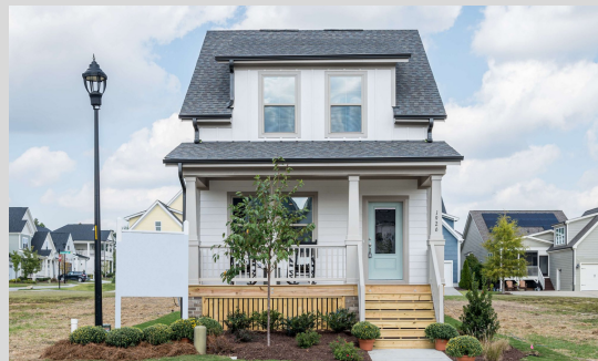
The Tiebreaker, Fresh Paint by Garman
