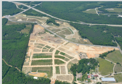
Progress on Phase 10 and The Collective (c/o Sanford Contractors)
